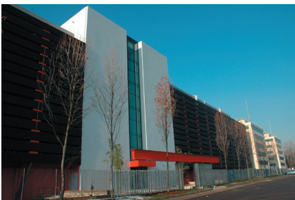
The state-of-the-art building features an innovative energy efficient water-cooling system
